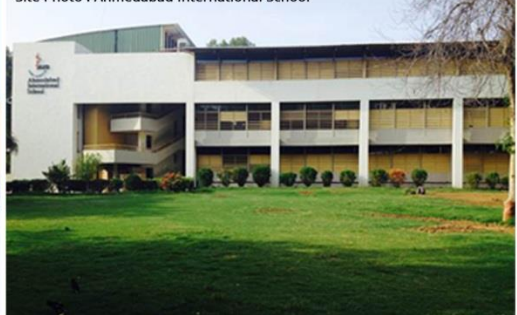
Site Photo : Ahmedabad International School
